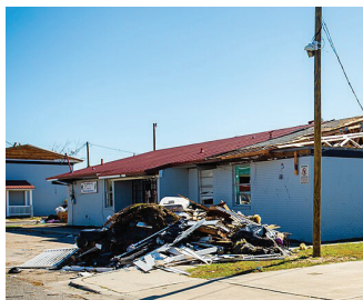
Florida panhandle following Hurricane Michael
