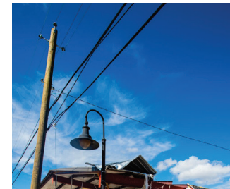
Florida panhandle following Hurricane Michael
