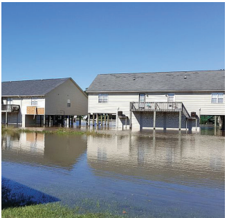
Hurricane Matthew Aftermath Greenville, NC Flooding
