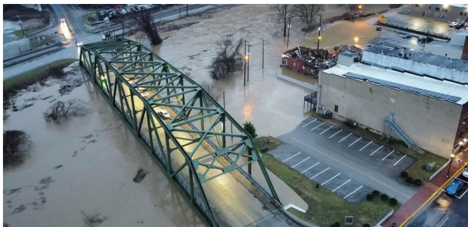
Image: Flooding in downtown Hazard, Kentucky, Feb. 15, 2025
